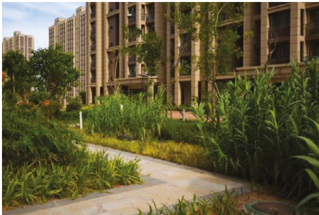
Sponge City's permeable pavements help reduce run-off
