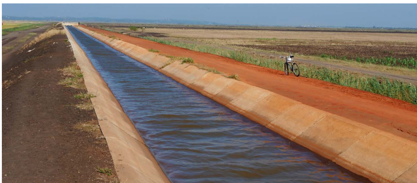
The Baixo Limpopo Irrigation and Climate Resilience Project in Mozambique
