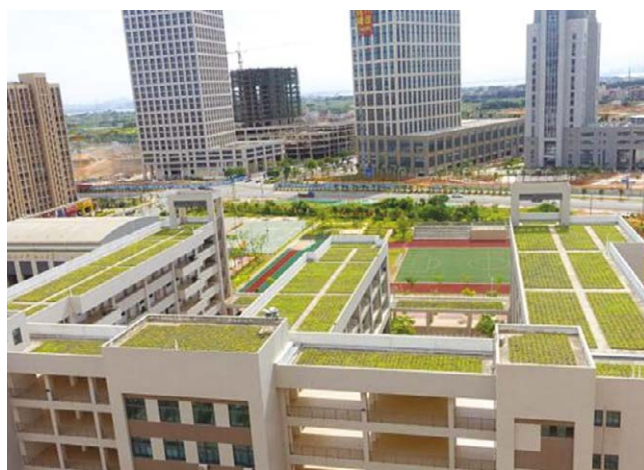
Green roofs and rainwater collection tanks, which store water for reuse
