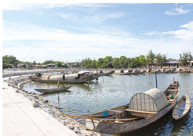
Specially designed dykes offer shelter for up to 100 fishing boats from damage during floods and typhoons, hence protecting local fishing folks' main economic assets and securing their livelihood
